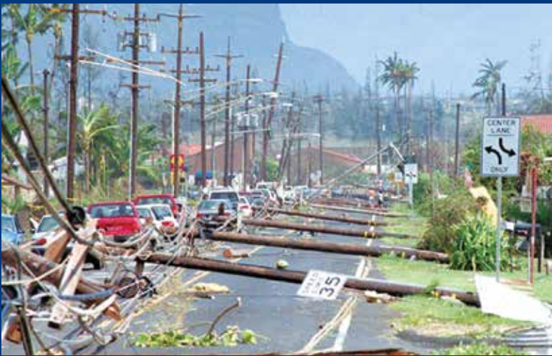
Hurricane Iniki damage, Kaua'i, 1992. Bruce Asato, Honolulu Star-Advertiser.
